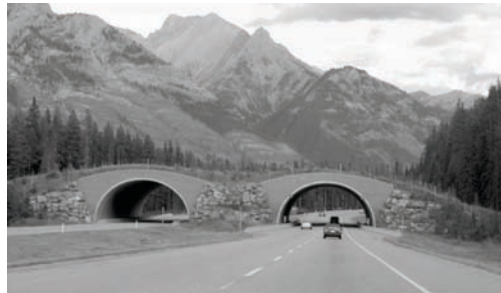
A Trans-Canada Highway 'wildlife crossing', one of many structures which successfully provide Yellowstone to Yukon connectivity conservation across an otherwise dangerous barrier for wildlife.
