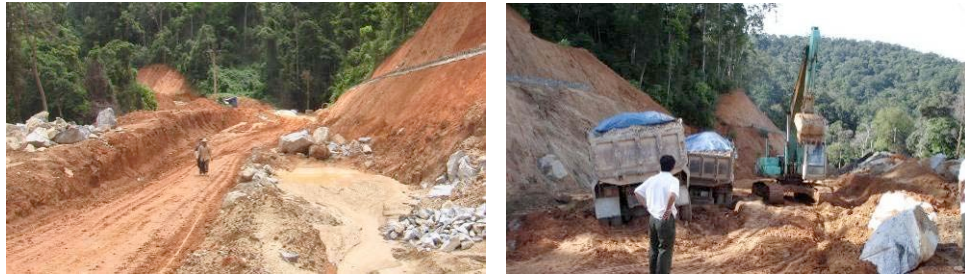
The East Truong Son Road under construction in the Green Corridor
